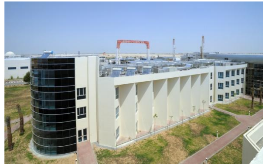
Image 1 – Elevated view of accommodation building
